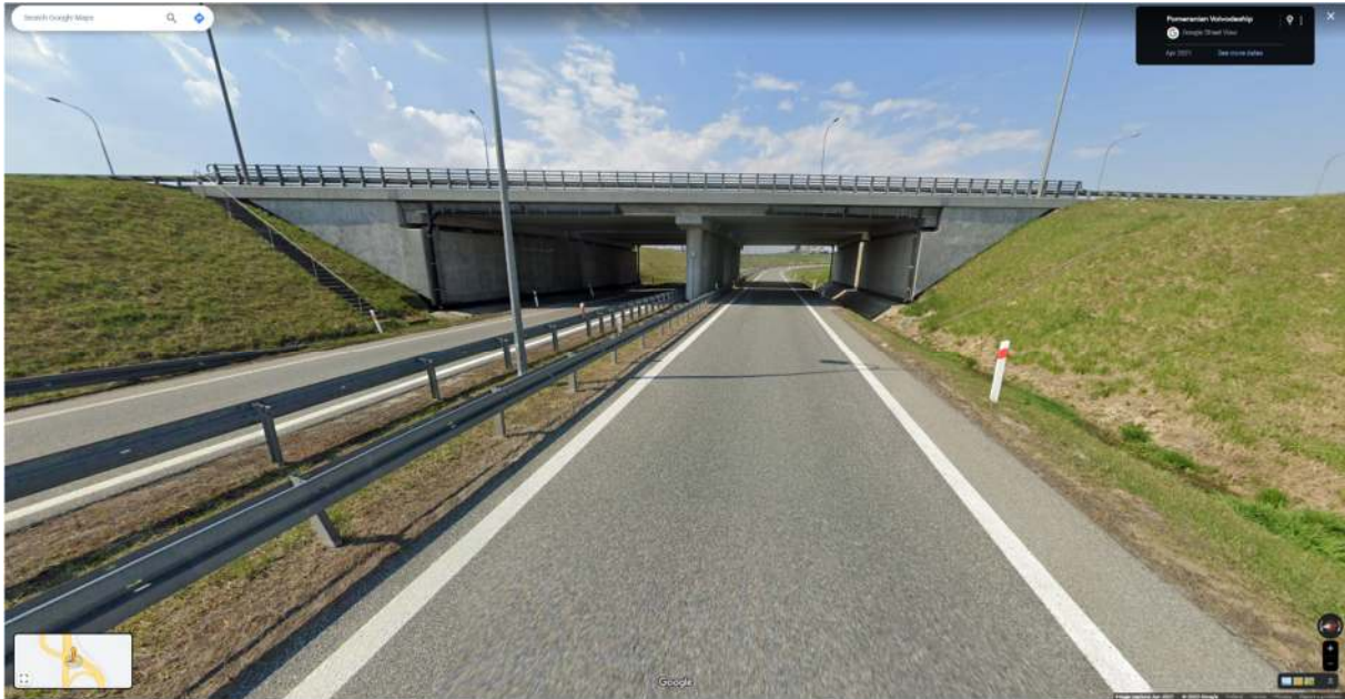
Figure 10. Interchange – Google Maps street view
